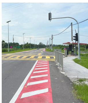
Thermoplastic Marking
